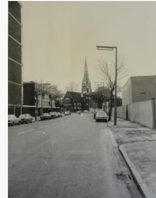
St. Edmund's RCC
